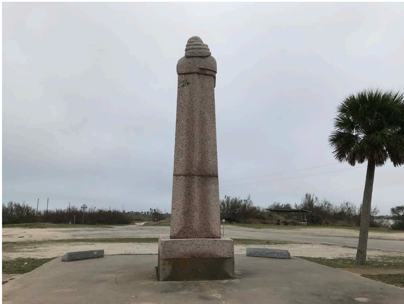
Photo 4: Rear (northwest) elevation of the La Salle Monument—camera faces southeast. The shaft is composed of four pieces, on which a combination of full-rounded and relief sculpture is carved.
