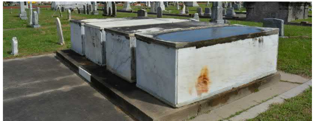
Crypts in a mausoleum and above grade vaults at Broadway Cemetery, Galveston County
