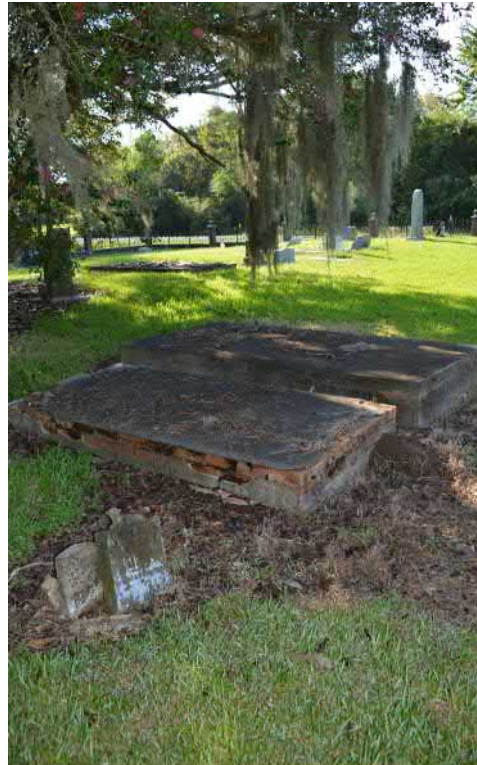
Brick and concrete vaults at Wallisville Cemetery
