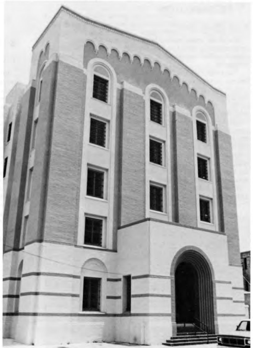
Old Bexar County Jail, San Antonio, TX. Renovated for use as offices in 1987. The developer benefitted from the city's policy of forgiving taxes on rehabbed historic properties. City of San Antonio photo; courtesy American Planning Association.
